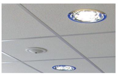
Thanks to its hemispherical lens, a single Q24M can monitor an entire room right into each of the four corners (360° Panorama View). The camera's should ideally be positioned on the ceiling in the center of the room. Due to its inherent physical and optical properties, the precision of the lens decreases as the distance from the lens grows. This means that the maximum
