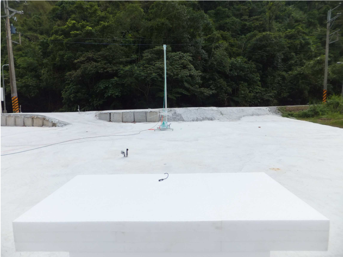
03 RE Front View
