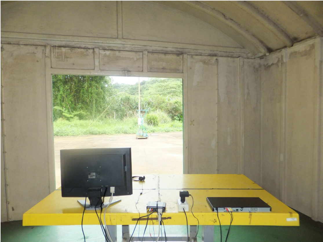
04 RE Rear View
