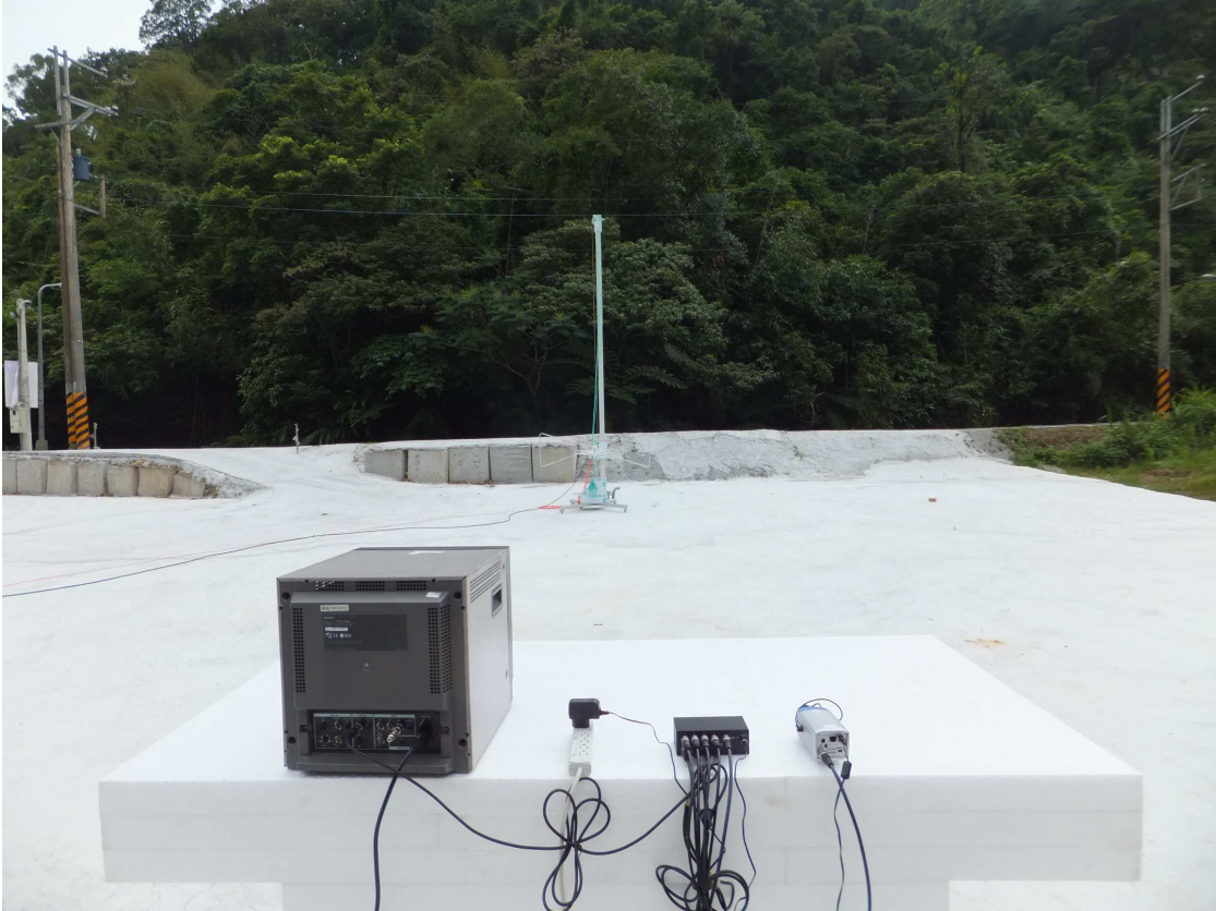
04 RE Rear View
